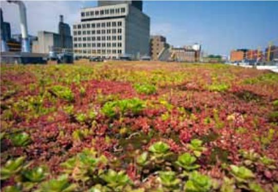
The vegetated roof on Montreal's Centre for Sustainable Development absorbs up to 23,000 litres of rainwater, reducing the incidence of wastewater overflows into the St. Lawrence River.<sup>2</sup>
